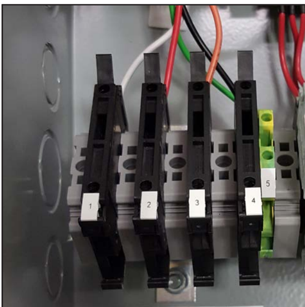
FIGURE 2 LC6000 Fused Power Supply Terminals
