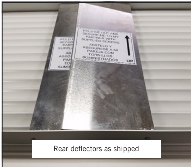
FIGURE 5 Fold-Out Diverter
