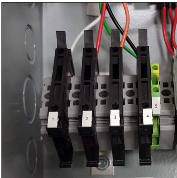
FIGURE 12 LC6000 Fused Power Supply Terminal
