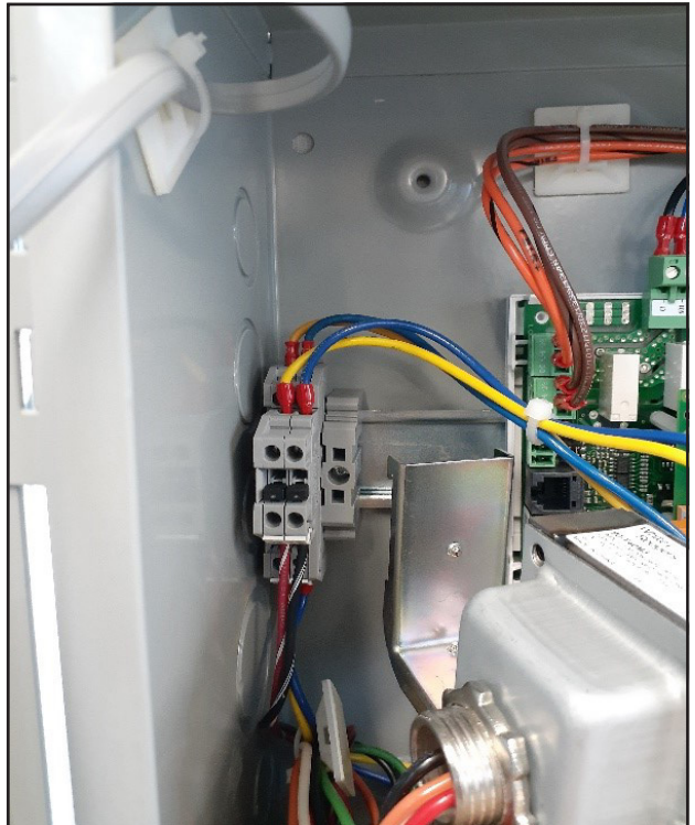
FIGURE 12 Transformer Removed
